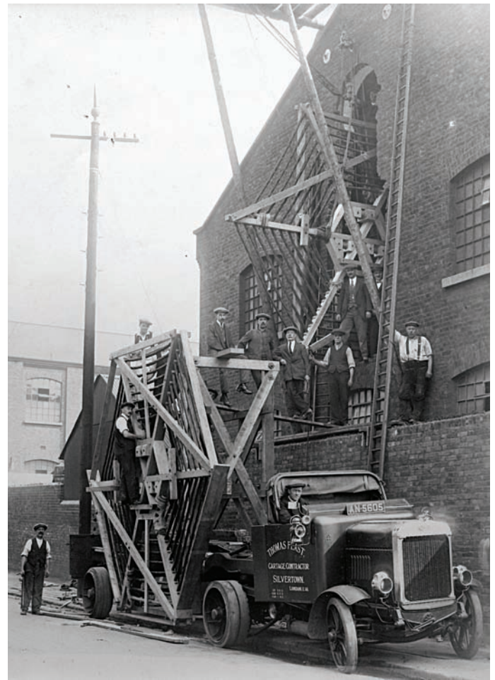
Above: The large size necessitated the demolition of part of the factory wall when it came to loading the spiders for delivery to Rugby.
