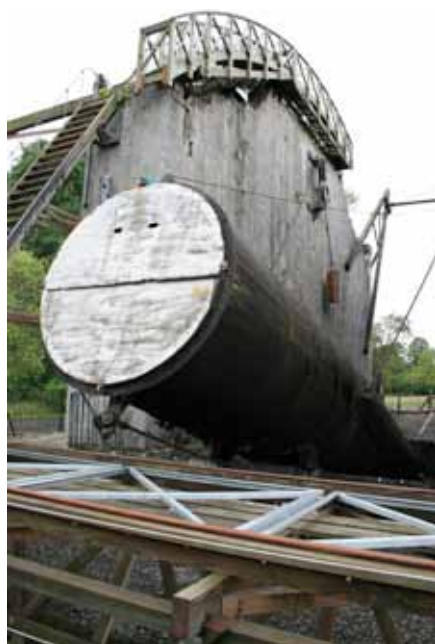
Two views of the massive masonry walls of the 72 inch telescope with the replacement tube and the complicated machinery and viewing platforms that were restored in the 1960s.
