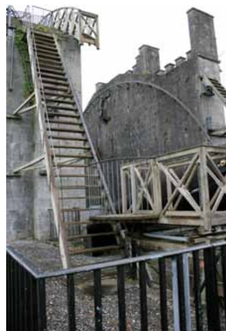
Two views of the massive masonry walls of the 72 inch telescope with the replacement tube and the complicated machinery and viewing platforms that were restored in the 1960s.
