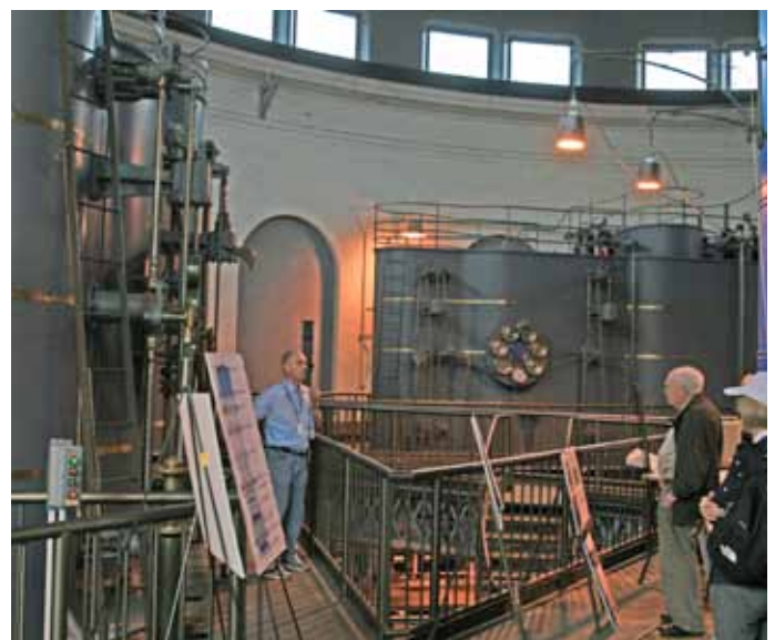
The waterworks engines with the steam cylinders in the background
