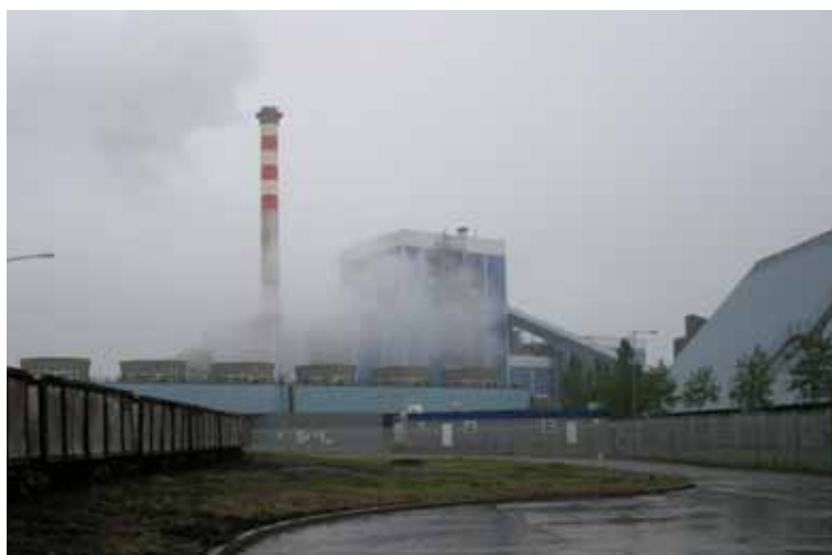
Edenberry Power Station
