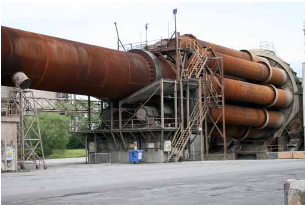
Below: A series of chemical reactions and heat of 2000°C turns the meal into cement clinker in the continuously rotating kiln
