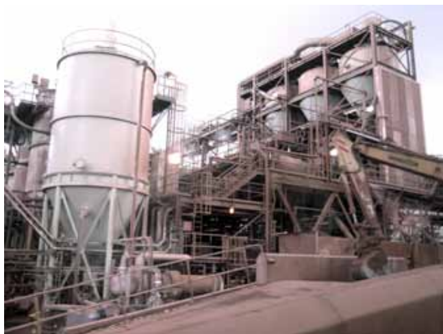
The separation of the sodium aluminate solution is done in two stages. First the sand is allowed to drop into large vessels.
