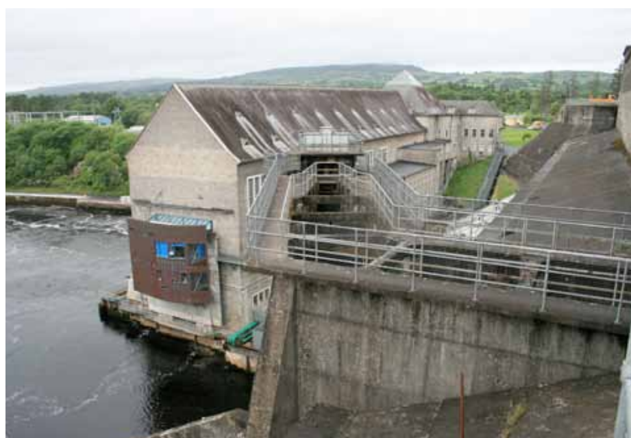
Another view of the power station showing the 1959 fish lift in the foreground
