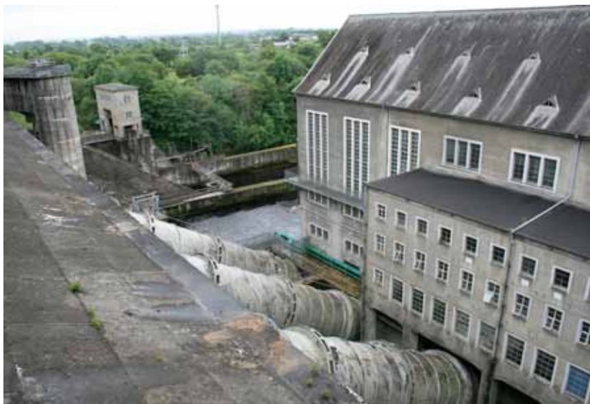
The power station showing the penstocks which carry water from the headrace to the turbines
