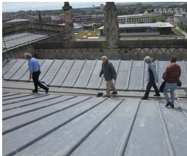
Crossing the roof to the central tower.
