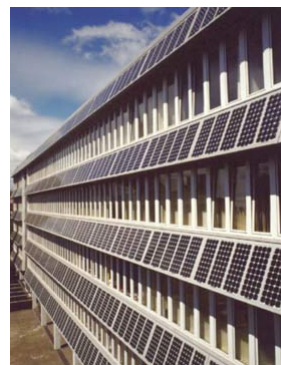
Northumbria University's Northumberland Building has the UK's first solar PV façade, operational since January 1995.
