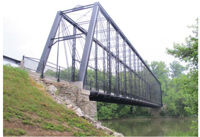
The Tripplle Whipple Bridge. Photograph: Clive Penfold.
