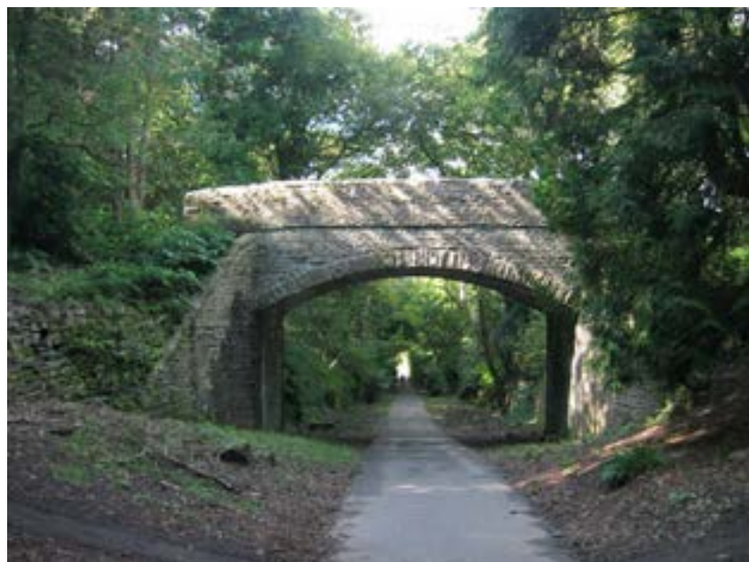
Robertstown cast iron tramroad bridge
