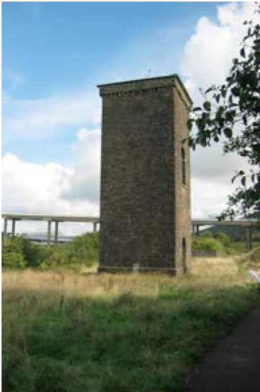
Hydraulic tower at Briton Ferry
