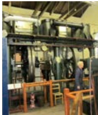
Worth Mackenzie triple expansion engine, inverted, condensing engine, installed 1895
