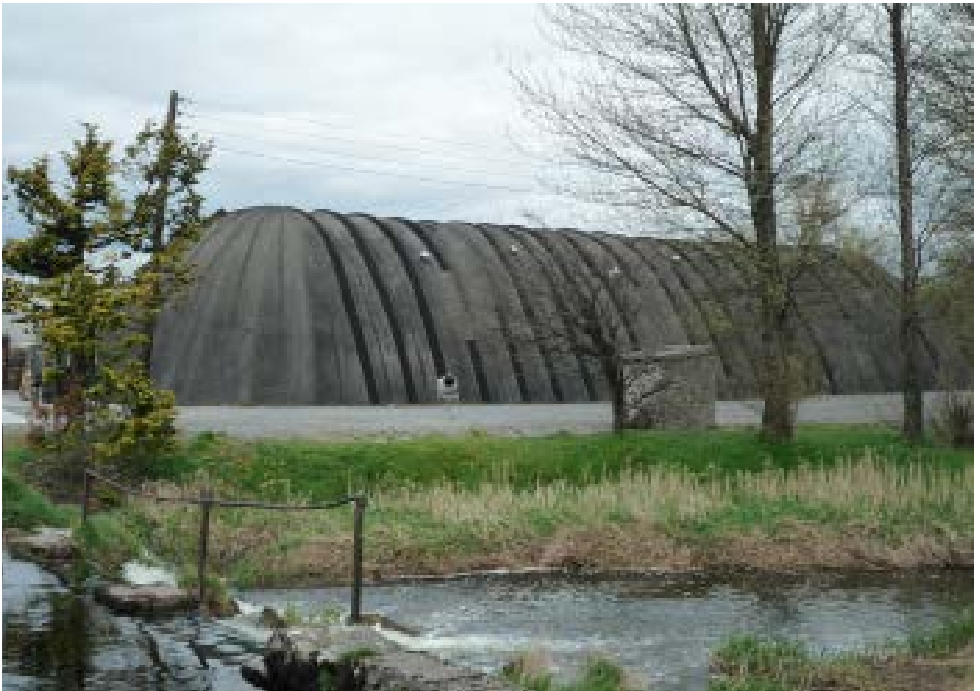
The Ctesiphon store at Locke's Distillery at Kilbeggan, Co. Westmeath in central Ireland
