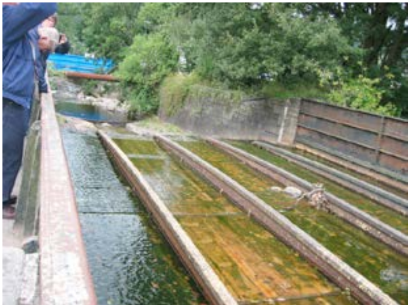
Brunel's cast iron aqueduct
