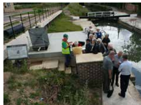
The group waiting to enter the turbine building alongside the rebuilt lock. All images: ©Mike Constable 2014.
