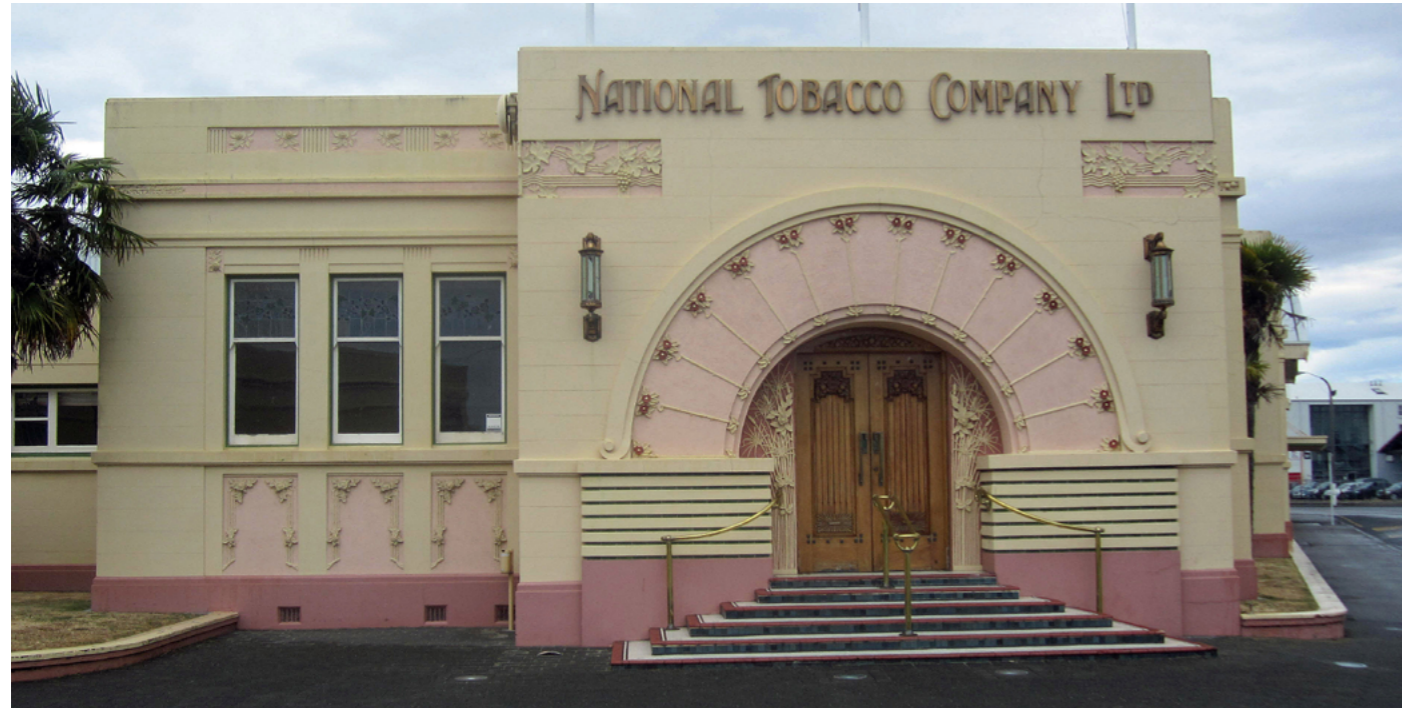
The Art Deco style National Tobacco Company Building in Napier Port was opened in 1933.
