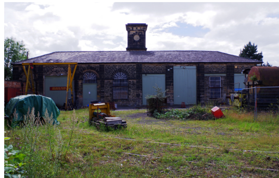
The former "Merchandise Station", a single storey goods shed completed by Thomas Storey in 1833. (image: Jonathan Aylen)
