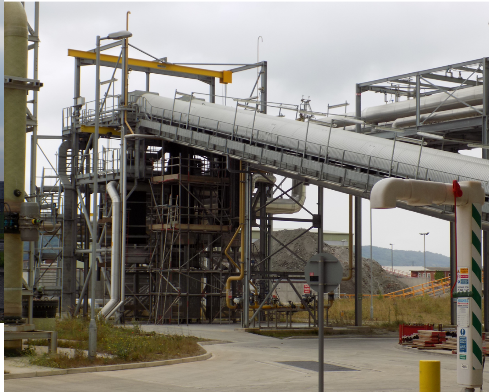
Energy from waste, conveyor system for bottom ash. Image: Jonathan Ayles
