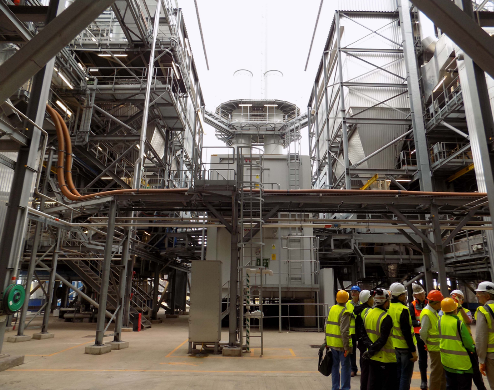
The crucial emissions filtration system and emission stack. Image: Jonathan Ayles
