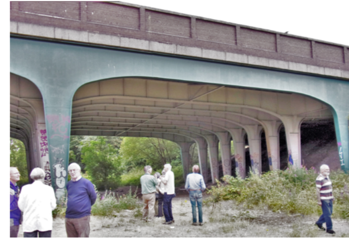
One of the 48 ft spans of the bridge. Charles Morris is in the centre of the picture. Image: Fred Starr
