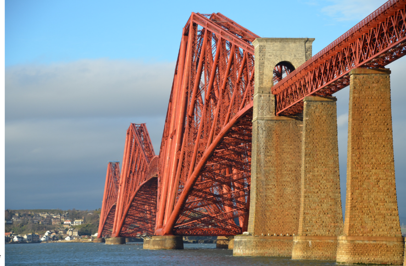
Forth (Rail) Bridge 1882-1890
