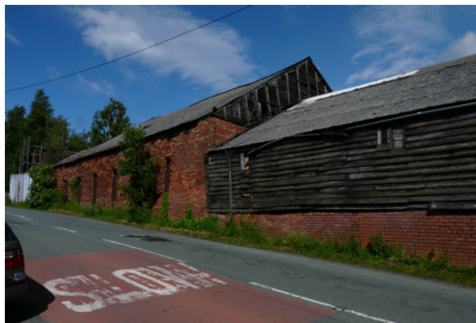
The Lion Salt Works before restoration. The restoration of Lion Salt Works was a formidable task as the area is prone to subsidence and the functional buildings were decaying.
