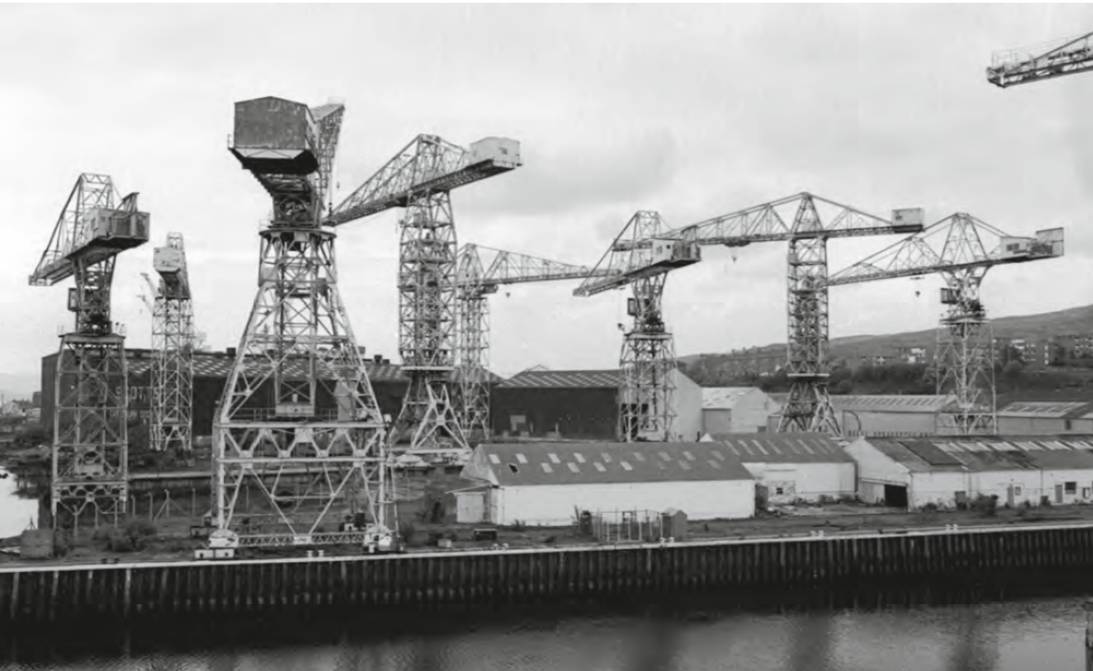
Cartsburn Shipyard, Greenock, showing Arrol cantilever cranes
