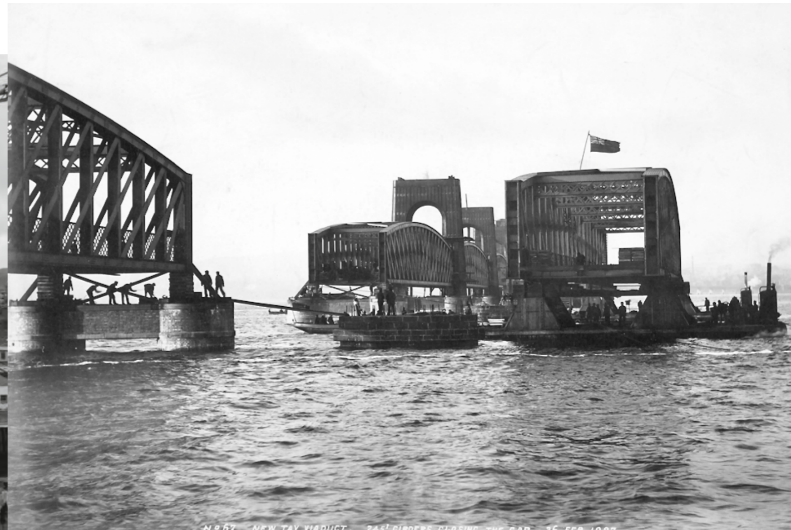
N 9,57 NEW TAY VIADUCT. 245' GIRDERS, CLOSING THE GAP. 26 FEB 1907.
