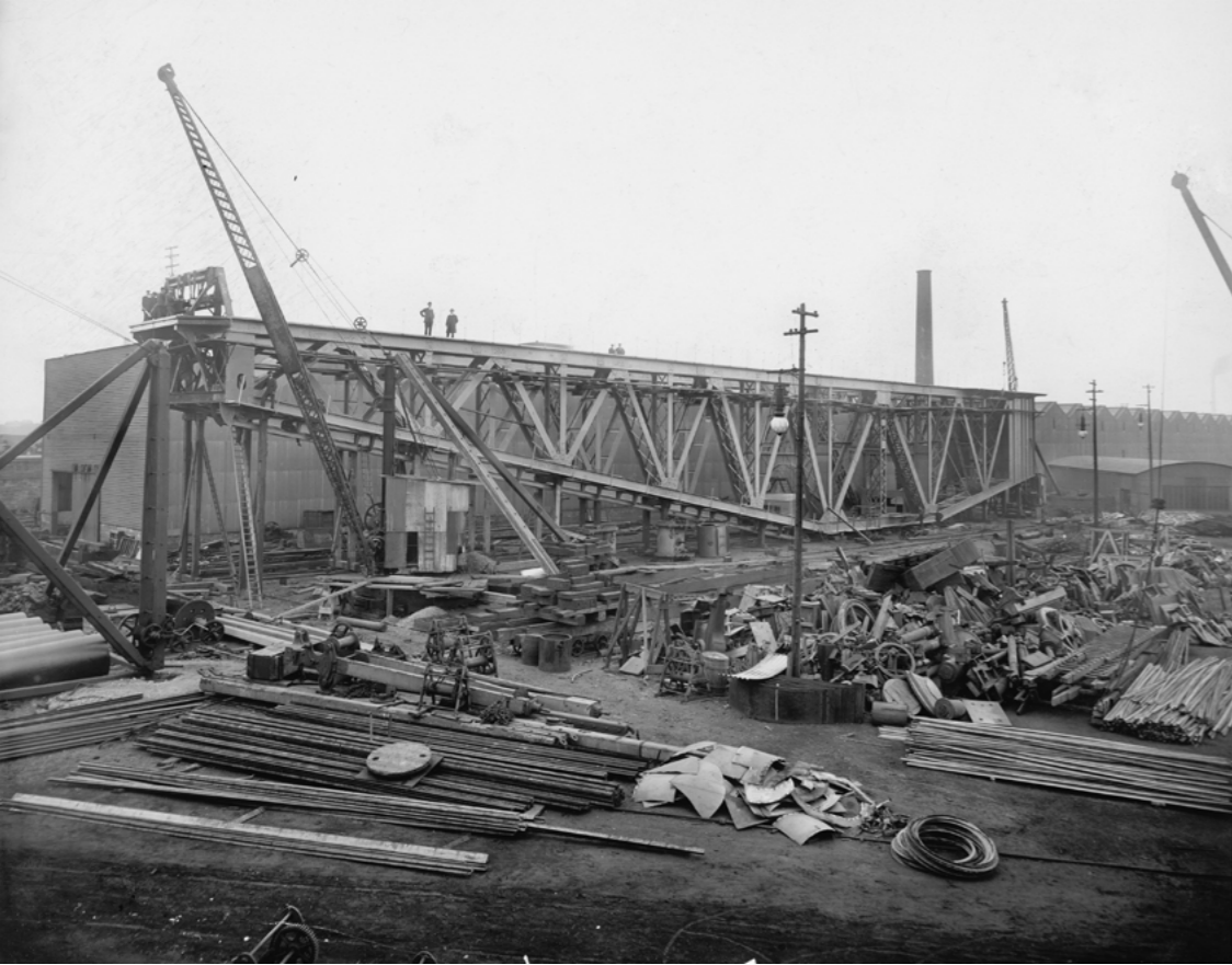
Construction of the Sasebo 250-ton Giant Cantilever Crane built by Arrol for the Japanese Imperial Navy in 1913, and still in operation
