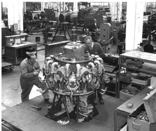
Figure 21. A Centaurus at Bristol in 1966 undergoing one of its infrequent overhauls.
